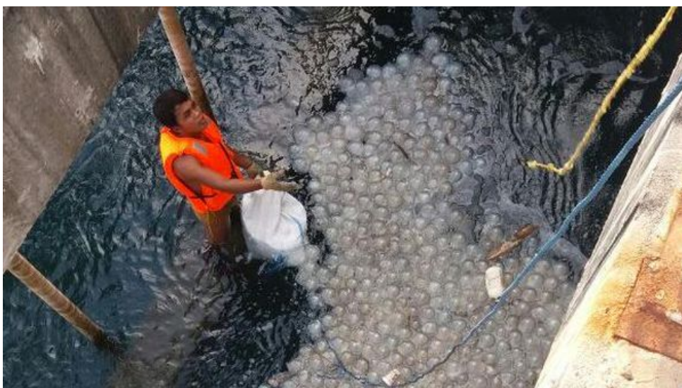
Fig 2.2.6 Jellyfish invading the cooling machine (Rofiq, 2016).
